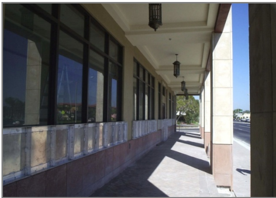
Example of Dry Flood Proofing removable panels utilized in a Bank Building in Naples Fl. – Appropriate in the Austin Street Corridor and Waterfront Overlay Districts.
