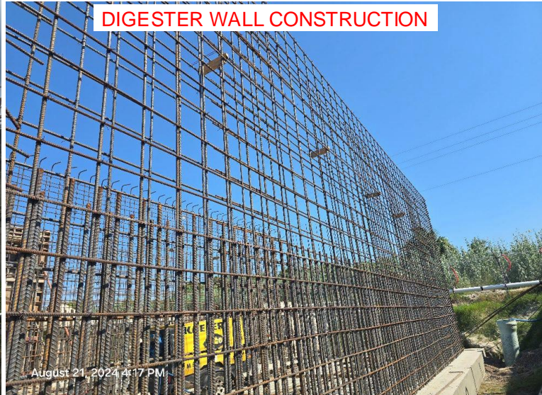
DIGESTER WALL CONSTRUCTION
