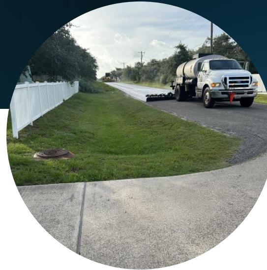
Each year, the City carries out its annual seal coat program to extend the life of our streets and keep them in good condition. Seal coating helps protect road surfaces from weather, water, and traffic wear, reducing the need for costly repairs in the future. This preventative maintenance keeps our streets safer, smoother, and more durable for everyone who travels through our community.
