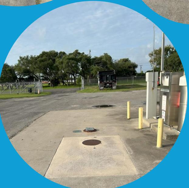
The City is removing its outdated unleaded and diesel underground fuel tanks in compliance with TCEQ requirements. Removing these tanks was important to eliminate potential environmental risks, ensure regulatory compliance, and reduce the liability associated with aging infrastructure. Fueling for City vehicles and equipment is now managed through the WEX fuel system, which provides improved accountability, tracking, and efficiency.
